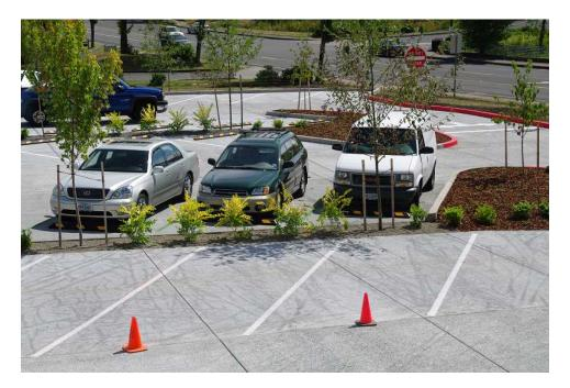
by: SUBMITTED PHOTO - New native plantings in linear tree wells work with vegetation bioswales, above, and newly installed porous concrete pavement to filter and minimize stormwater runoff in the Sunset Swim Center parking lot.
